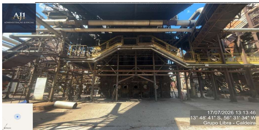
Figura 2 – Caldeira A Lenha/Bagaco De Cana 01 Retangular Dim 8000x8000x20000 Mm Cap 9000
