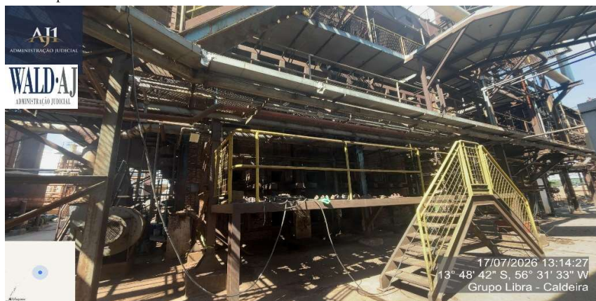
Figura 3 – Caldeira A Lenha/Bagaco De Cana 02 Retangular Dim 8000x8000x20000 Mm Cap 130000.
