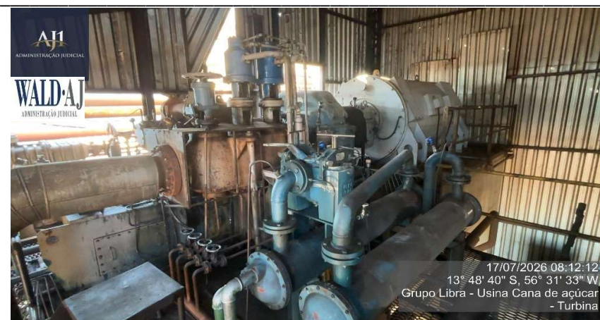
Figura 20 – turbina cap 4000 kw mca dedini mod dme-450 b
