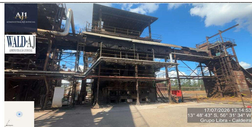
Figura 4 – Caldeira A Lenha/Bagaco De Cana 03 Retangular Dim 8000x8000x20000 Mm Cap 45000
